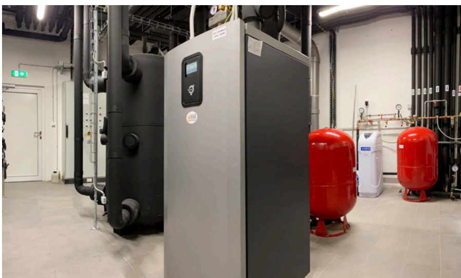
Machine room with Thermia Mega
